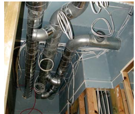
(top right) Sections of three trusses that had longitudinal splits were wrapped in airtight membrane, then additionally protected with OSB boxes; ductwork for the MVHR system
