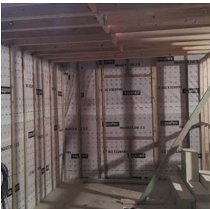
(above, from top) Wood fibre insulation board, fixed directly to the existing wall, was selected primarily for moisture management properties; followed internally by the timber frame with more wood fibre insulation; and then by an airtight vapour barrier; condensation risk was assessed with Wufi, including this simulation of moisture content in the insulation layer with 100mm Pavadentro + Pavatex DB 3,5 + 80mm Pavaflex between studs on the south west elevation
